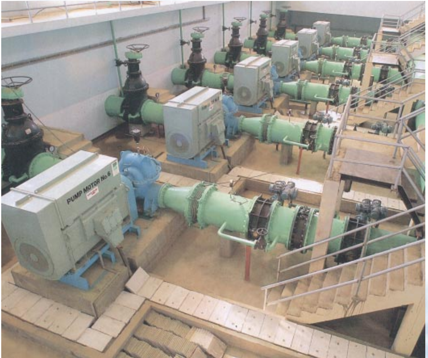
Horizontal Split Case pumps and Butterfly valves at Gujarat water supply and sewerage board, Pipli, Gujarat
