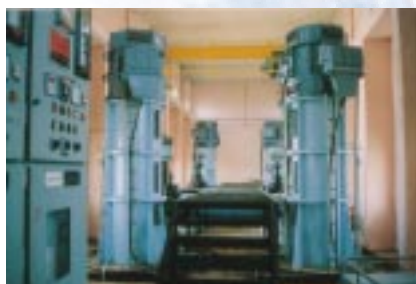
Vertical Turbine pumps installed at Ichalkaranji Water Supply Scheme, Dist. Kolhapur
