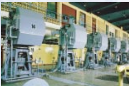
Vertical Turbine pumps installed at Pise pumping station, Mumbai.
