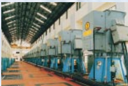
Vertical Turbine pumps installed at Mhaisai Lift Irrigation Scheme, Sangli
