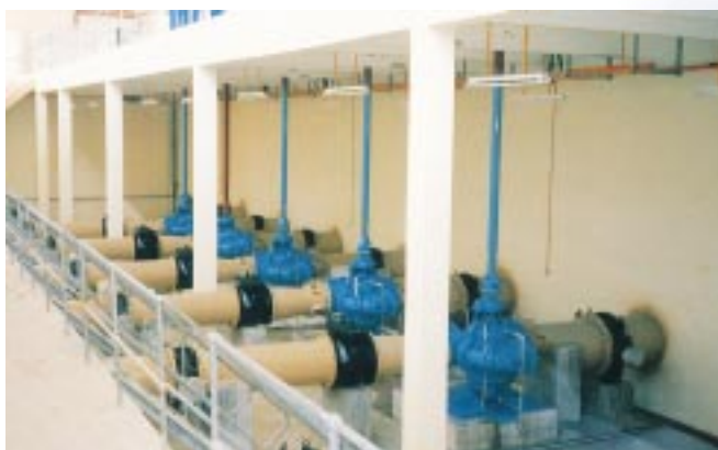
Axially Split Case pumps in vertical execution, for a water supply scheme in Kedah, Malaysia
