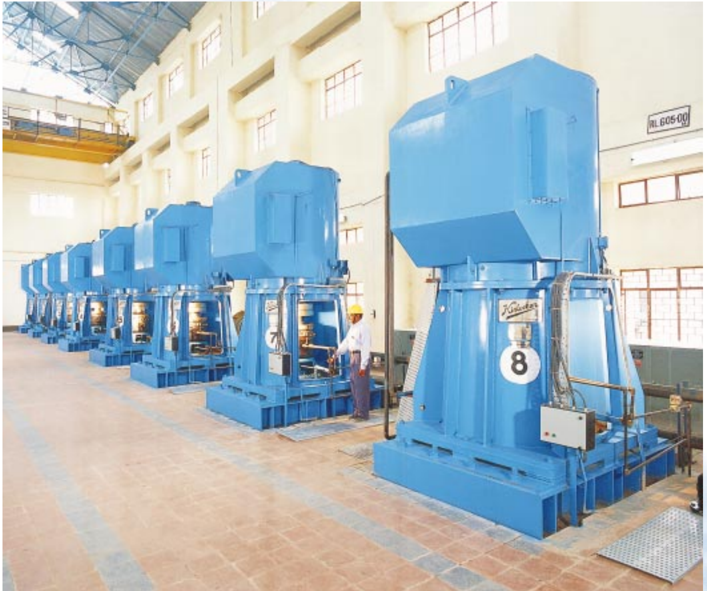
A series of Vertical Turbine pumps at Takari in Maharashtra, for Irrigation purpose
