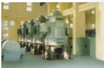
Vertical Turbine pumps installed at Koil Lift Irrigation Scheme, Padampura/Pulwana Srinagar
