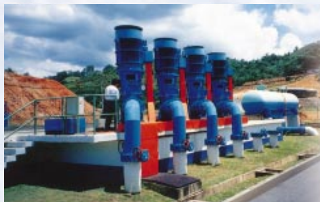
Vertical Turbine pumps in operation for a water supply scheme at Sabah, East Malaysia
