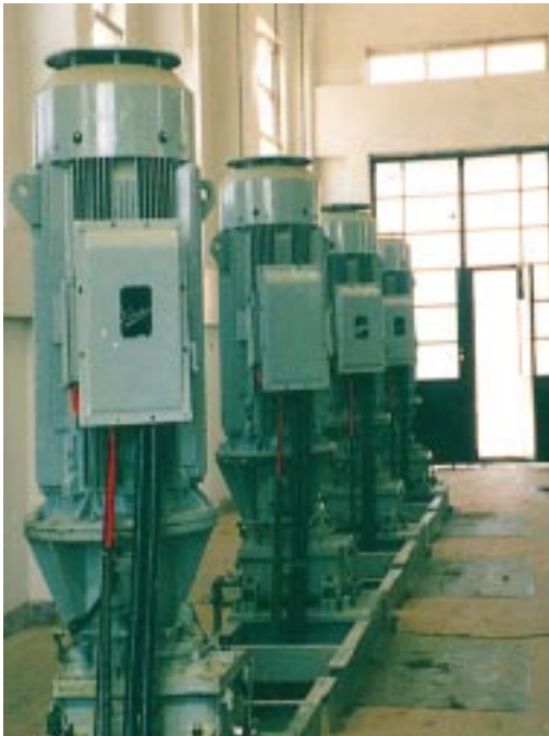
Vertical Turbine pumps installed for irrigation at Wadi Sheeh, Egypt
