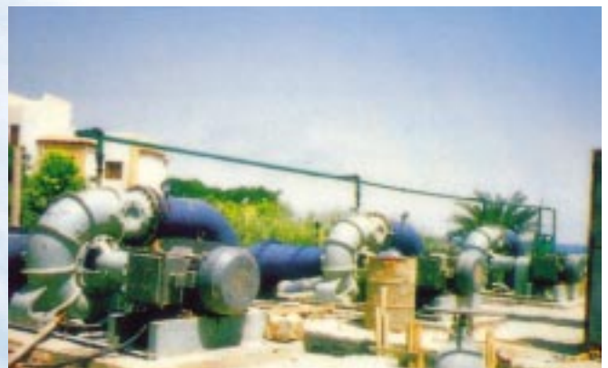
Mixed Flow pumps for sewage application at Faiyad Egypt.
