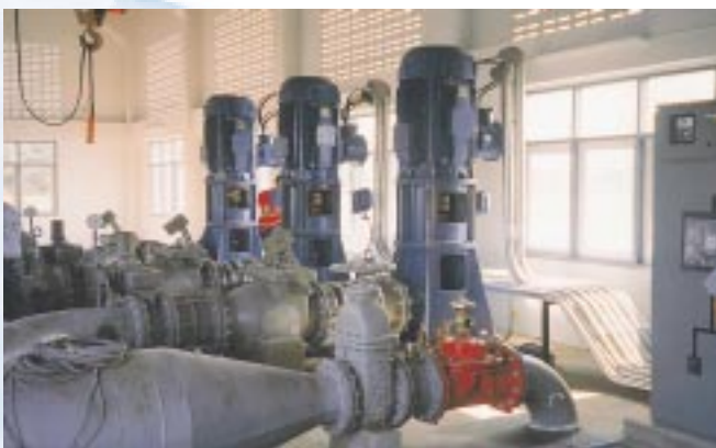
Vertical Turbine pumps in operation at Royal Bangkok irrigation scheme, Thailand
