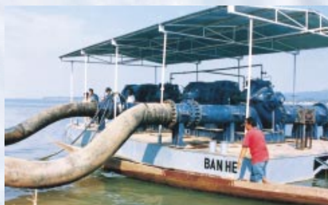
Split Case pumps at Banhe Pumping Station, Lao PDR
