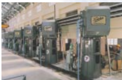
A Series of Vertical Turbine pumps and valves installed at Janai Sirsai Lift Irrigation Project, Pune.
