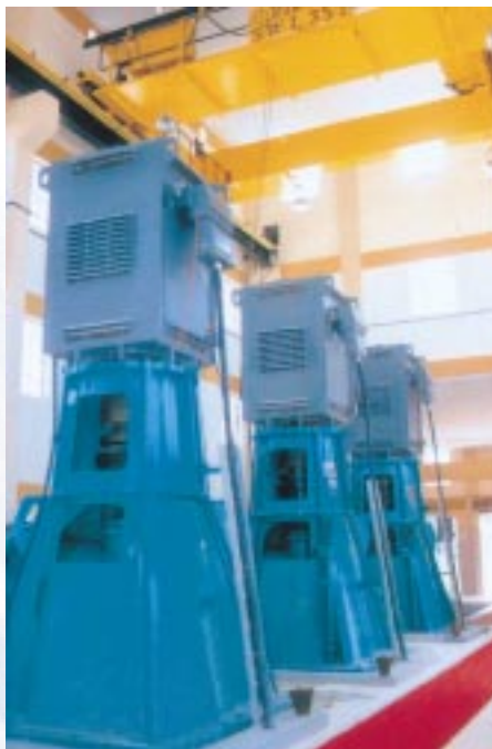
Vertical Turbine pumps installed at Chagalnadu Lift Irrigation Scheme, Andhra Pradesh.
